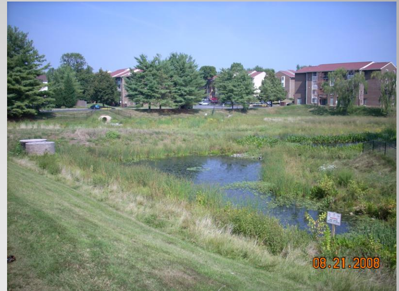
Dry Pond Converted to a Wet Pond. Peppertree Farms. Treated 38.4 Impervious Acres
