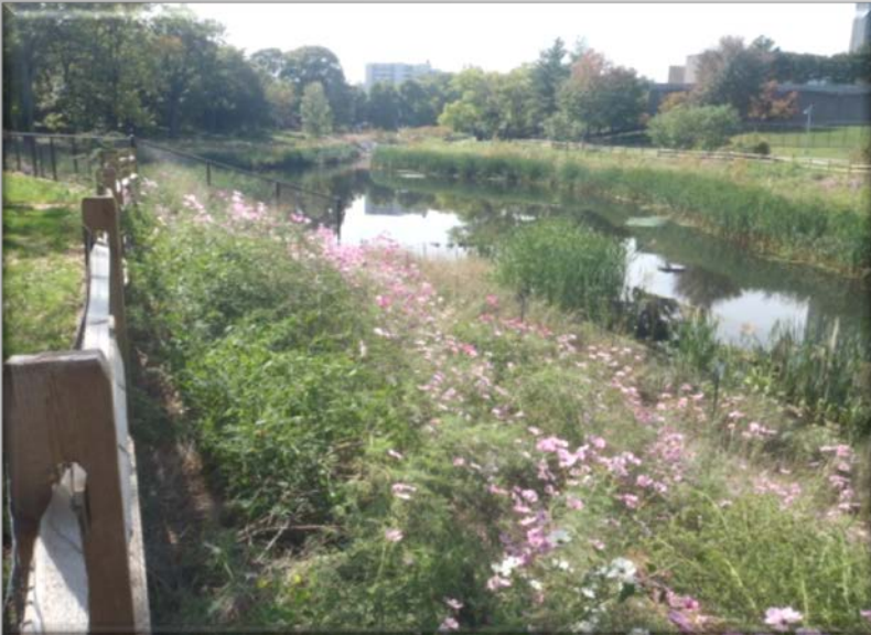
New SWM Pond, NIH, Treated 112 Impervious Acres
