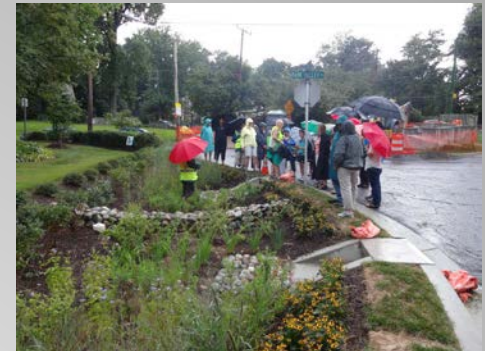
Bioretention in the Right of Way, Sligo Park Hills
