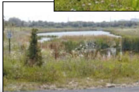
Constructed wetland in the Bailey Brook watershed helps treat runoff from the roads and parking lots.
