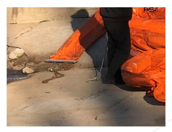
Chain used to connect boom cable to anchoring points. A come-along used to release boom from boat anchor point, once secured to VA shore anchor.
