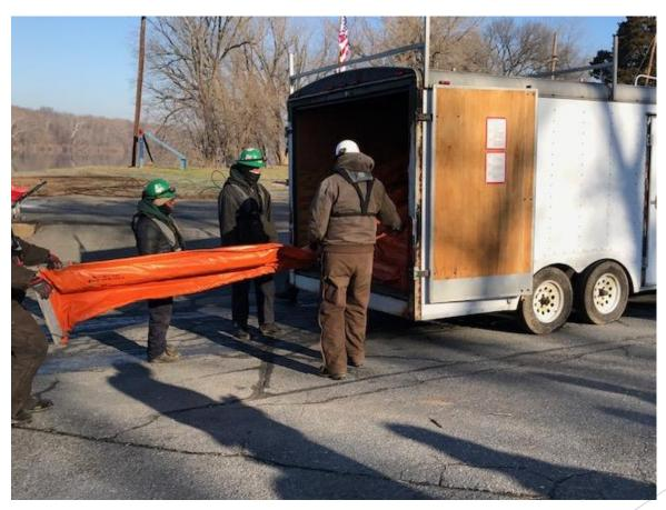
Unload all boom rather than flake from trailer. If not, any snag may drag trailer into water once ferry begins to pull boom across river.
