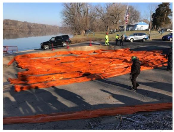
Ensure no cross overs; cables on top and bottom of boom must remain parallel and not twist once in water.
