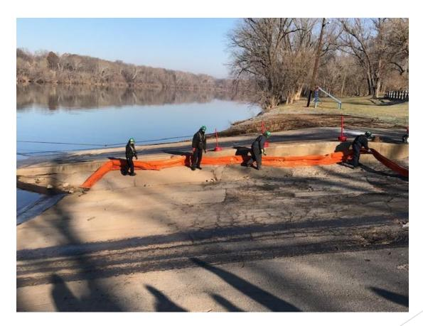
Next, bring VA end closest to boat, leaving enough slack to load extra to pull from secured anchor on boat to VA side land anchor.
