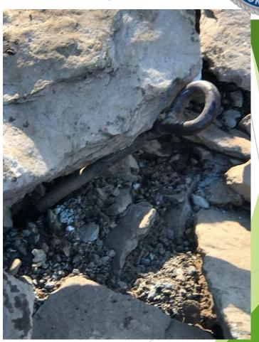
(left) Anchor point (MD) pulled out of ground, (right) and barely held for lower cable anchor
