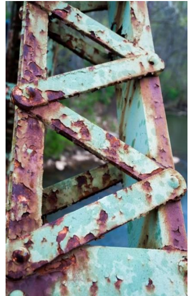
Bridge corrosion Photo by Jim Palmer.
